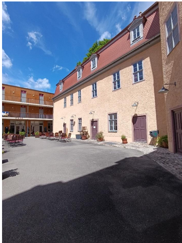
Figure 4: Courtyard of the Erbenhof (right). This is the concert area.
