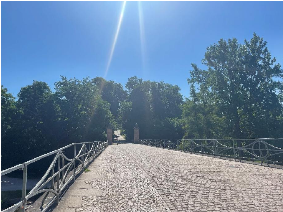
Figure 5: Entrance with stairs: “Sternbrücke”.
